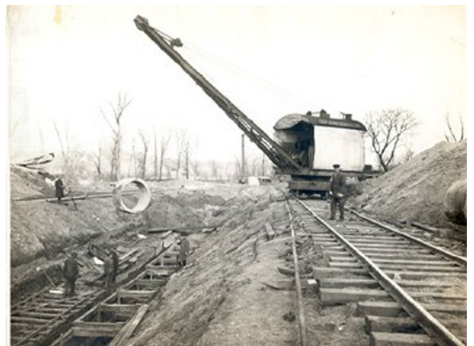
Construction of the Infiltration Gallery
